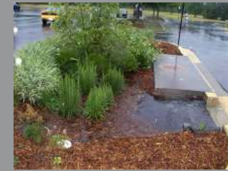
Storm water sump for landscaping
